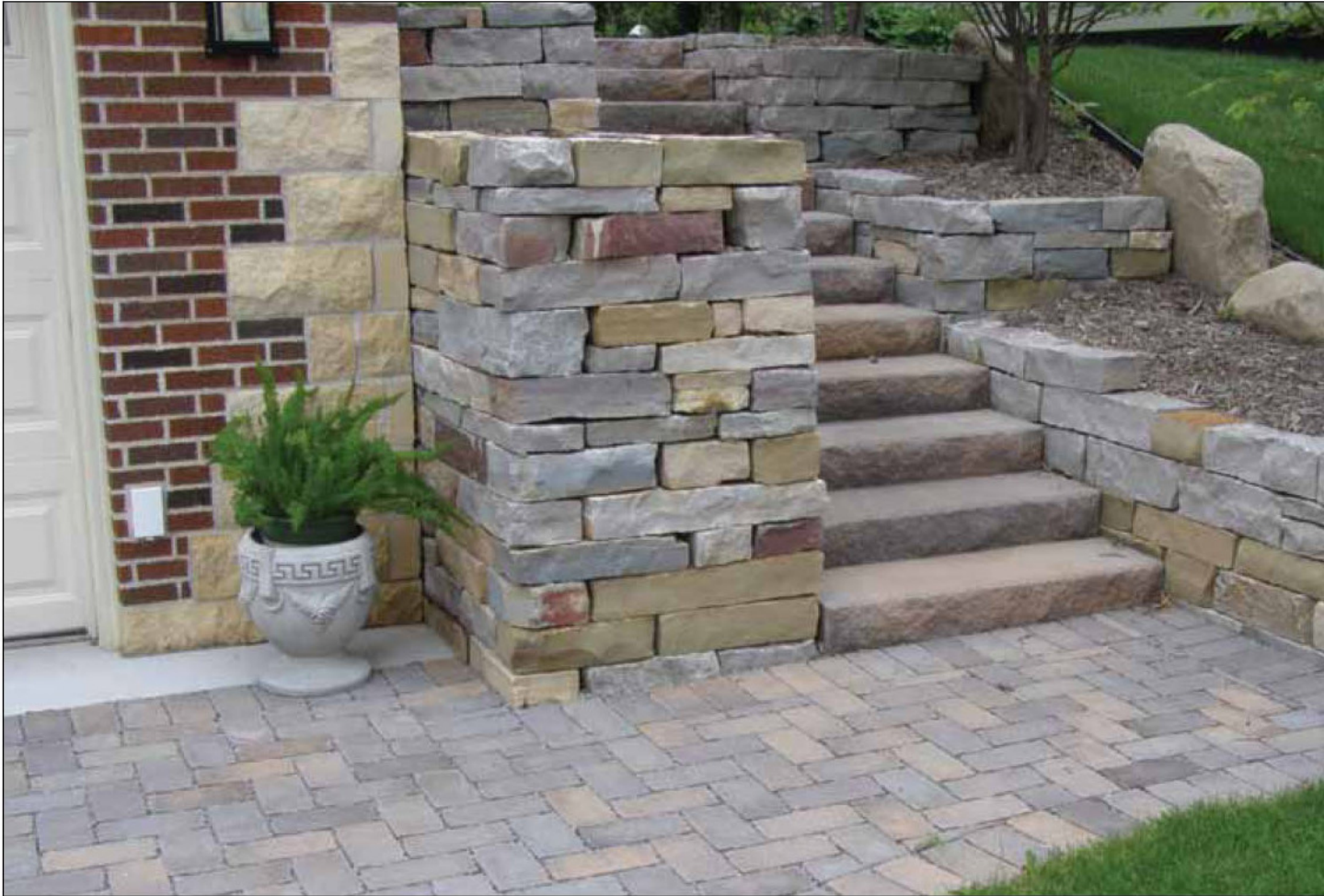
» Borgert Products concrete Step Units work with the natural stone walls at about $100 less (each) than the stone steps on the other side.
